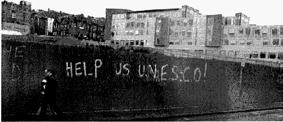
Nov '08 the New Street Gap Site hoardings, the CEC headquarters to right with Canongate Venture to rear
