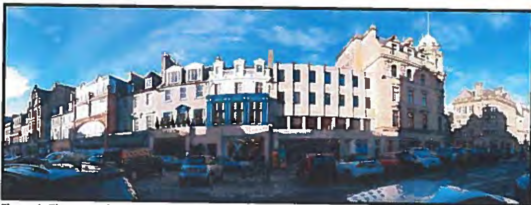
Figure 1. The street frontage around the application premises
