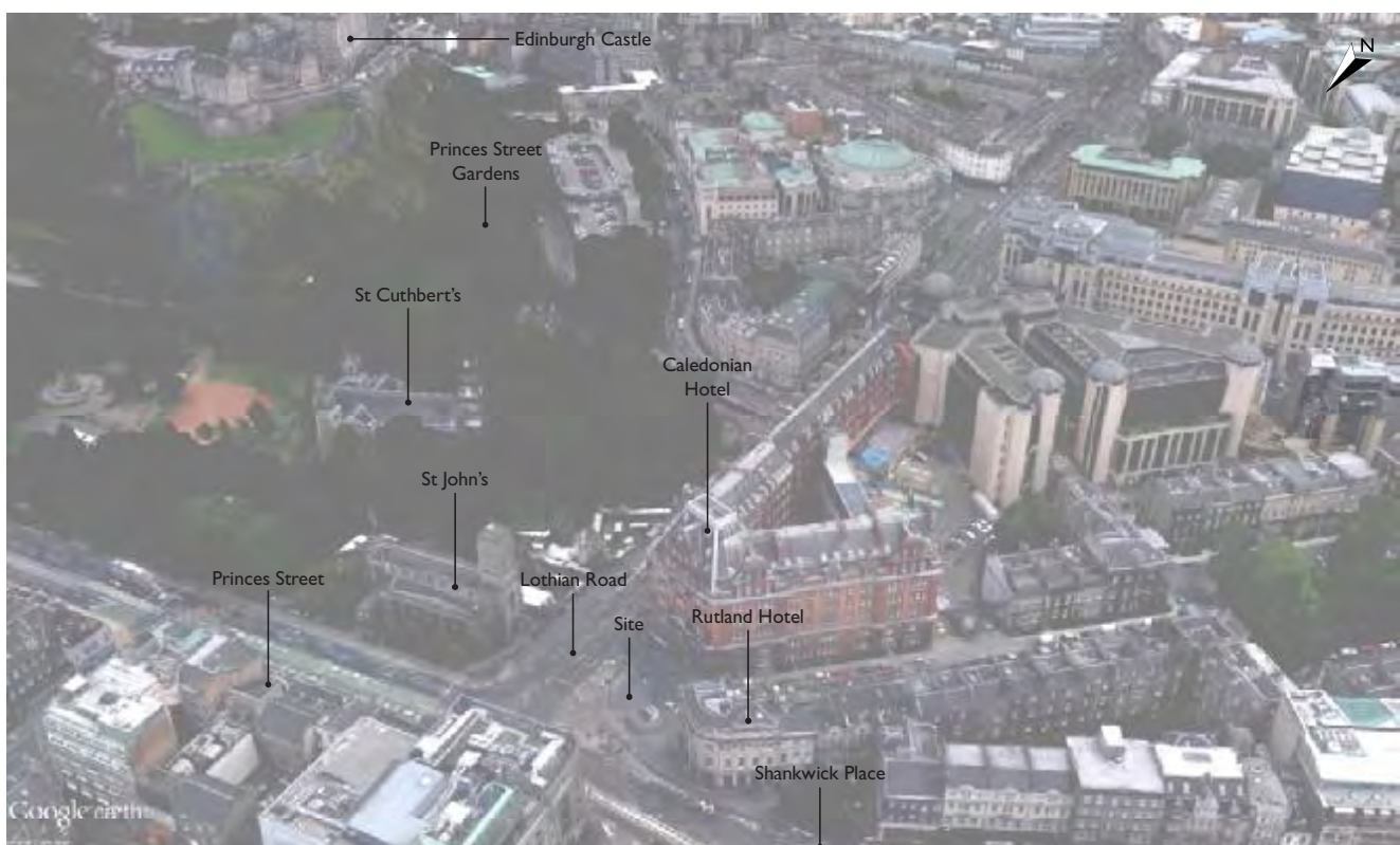
Aerial view of Edinburgh showing the location of key sites related to the Rutland Street proposals. Baseplan © 2016 Infoterra Ltd & Bluesky
