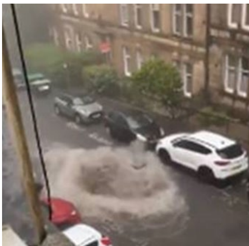
Example: Surcharging Sewer System at Capacity
