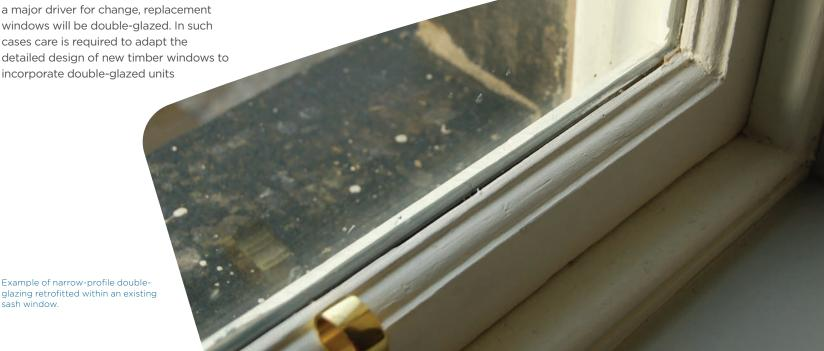
Some manufacturers have attempted to address this by using a standard double-glazed unit with applied astragals or an astragal cassette, often in conjunction with integral dividers in the cavity. Such approaches may be considered in cases where a replacement window will improve the current situation, allowing an aesthetically accurate match. Astragals sandwiched between panes alone, will be very unlikely to be acceptable.
