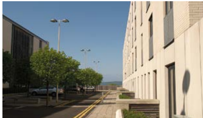
This new housing at Saltire Street in the masterplanned area has a view to the sea.
