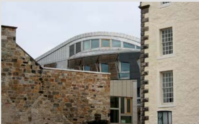
Metal roofing in a historic context—Canongate Stainless Steel roofing has been used on the Scottish Parliament.
