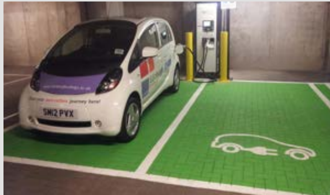
Fountain Park installation of underground car-park electric vehicle charging.
