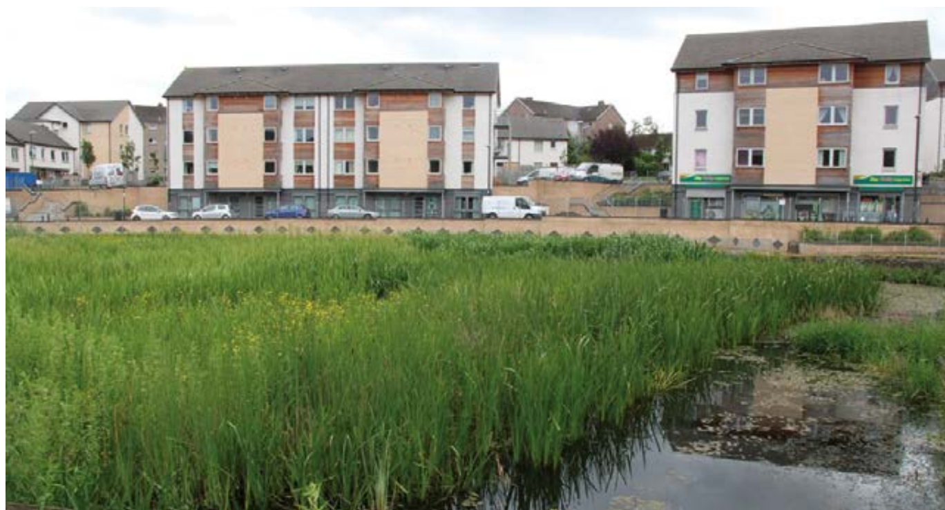
SUDS retention basin, Firrhill Neuk, Oxgangs
