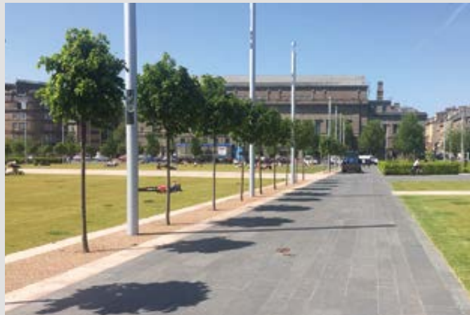
Dundee Waterfront Use of a continuous tree trench and underground cellular system to support surrounding paving surfaces as part of advanced green infrastructure at Dundee Waterfront.
