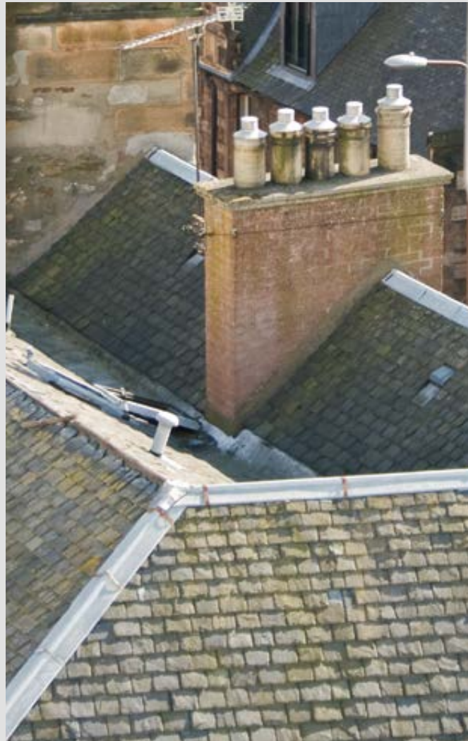
Traditional roofing materials (right) Slate, Lead and zinc are traditional roofing materials used in Edinburgh—seen here from the Museum of Scotland’s roof.
