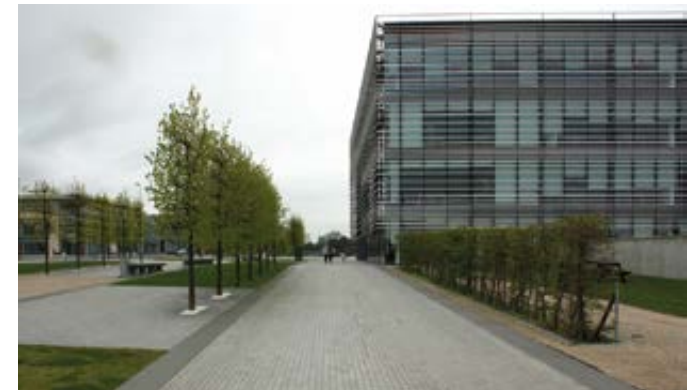
The office at Waterfront Avenue has a square in front and the space for a future public transport hub.
