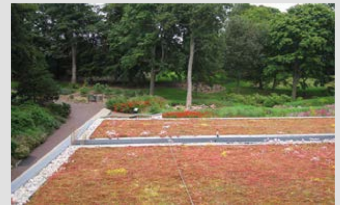
Extensively green roof—Botanic Gardens The planting on this green roof helps integrate the building into its surroundings.
