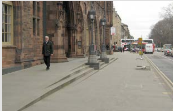
Queen Street New Town In the New Town, sandstone should be used as the paving material. The paving outside the Scottish National Portrait Gallery provides a model that should be used elsewhere in the New Town.
