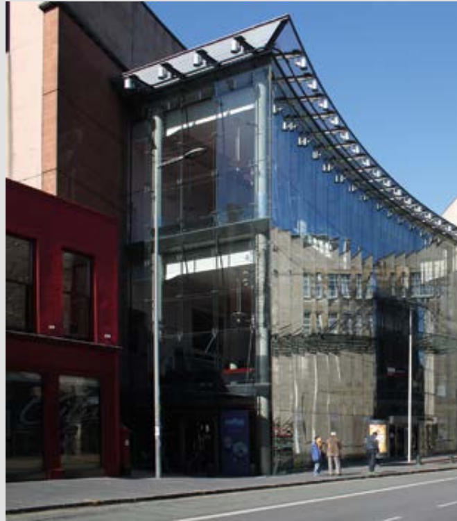
Frameless glazing—Festival Theatre, Nicolson Street The refined detailing of the frameless glazing helps create a striking modern addition to the street.
