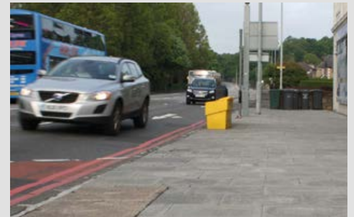
Western Corner Areas with significant footfall In other areas with significant footfall, such as local centres outwith conservation areas, rectangular precast concrete slabs (coloured grey) should be used.
