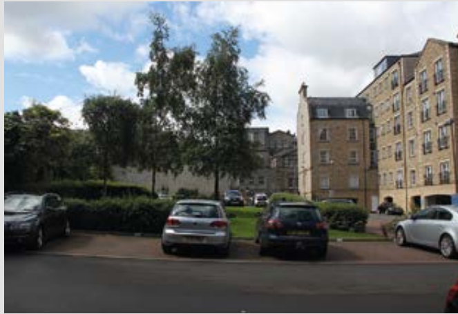
Rear courtyard parking within well overlooked landscaped amenity space off Gayfield Square
