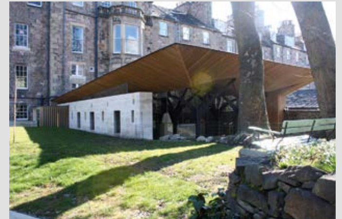
Frameless glazing—George Square Lane Glazing is used to create the effect of a floating roof on this building.
