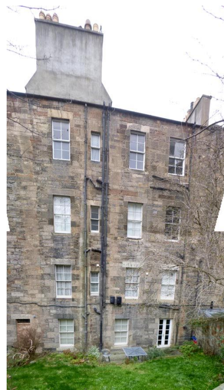
REAR ELEVATION PHOTO
