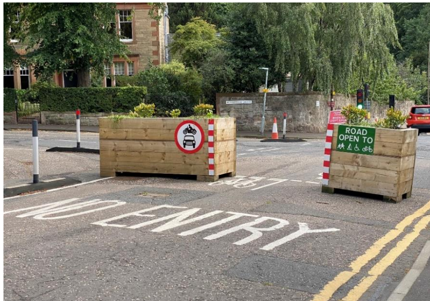
A modal filter implemented using planters restricting motorised traffic from entering or exiting Braid Road north of Hermitage Drive.
