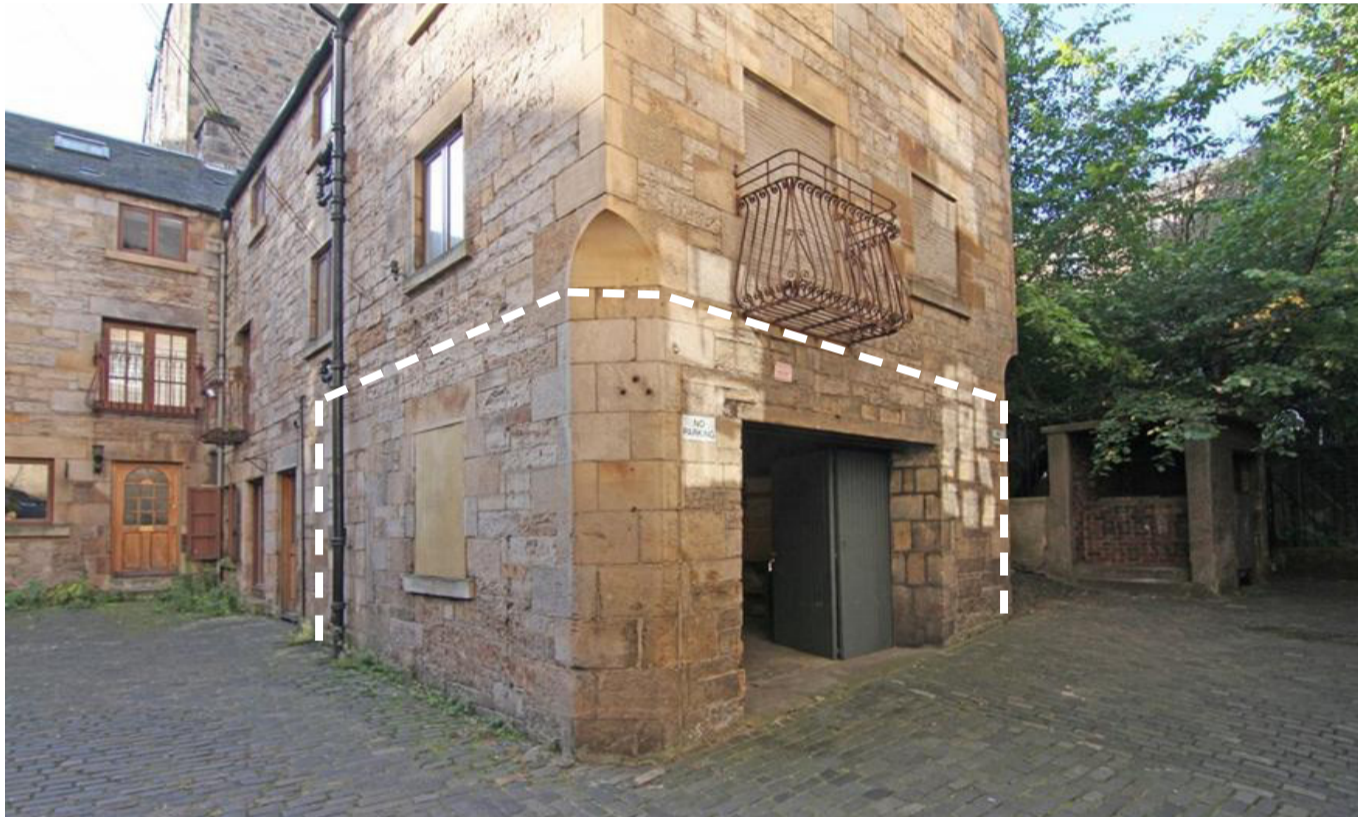
Photograph of North and East Elevations
