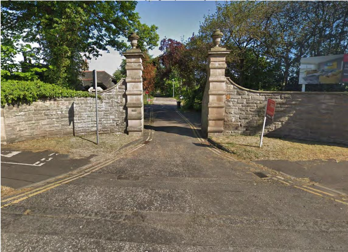
The width between the two piers was measured as 3.6metres. An existing priority system is in place to facilitate the managed two-way movement of traffic. Priority is given to traffic entering from the A8, ensuring there is no queueing back onto this strategic road.
