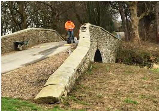
**Figure 20** The bridge, prior to restoration work, showing unstable coping stones
