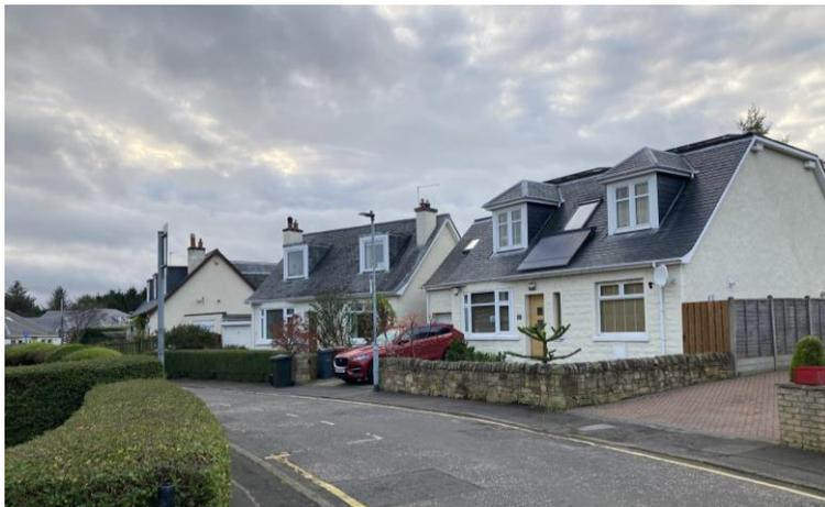
Figure 2 - 3 Craigleith Hill Green, pitched roof with 2 no. front dormers.
