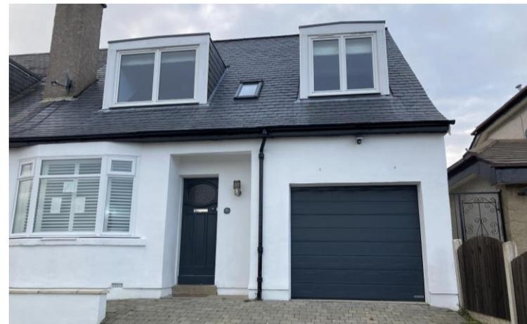
Figure 4 - 71 Craigleith Hill Crescent, pitched roof with 2 no. front dormers and widened roofline.
