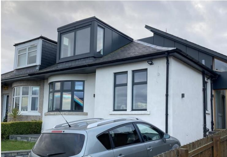
**Figure 9 - 59 Craigleith Hill Crescent, introduction of dormer window, increase in height and width of roofline.**
