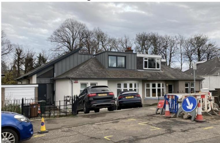
**Figure 10 - 7 Craigleith Hill Gardens – introduction of dormer window, increase in height and width of roofline.**
