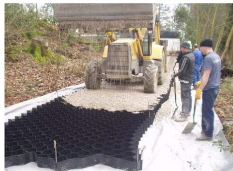
As well as avoiding disruption to the roots this reduces construction times and costs. It also prevents surface rutting, which increases the long-term performance and aesthetics of the final surface. The installation of a short section of this type of driveway is well-suited to this particular site, with no major differences in levels between the highway and the site.
