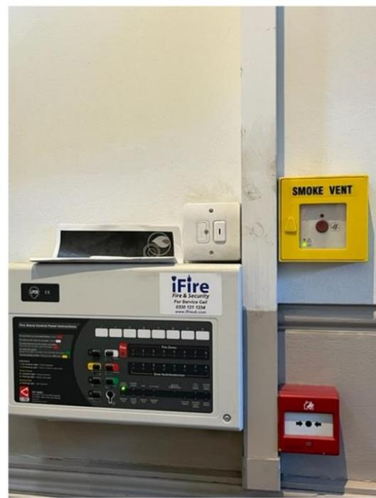
Figure 4. Central Fire Alarm System
