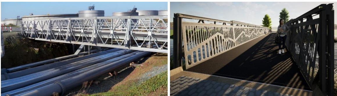
Figure 2 - Mabey Compact 200 steel modular bridge (Option 1)
