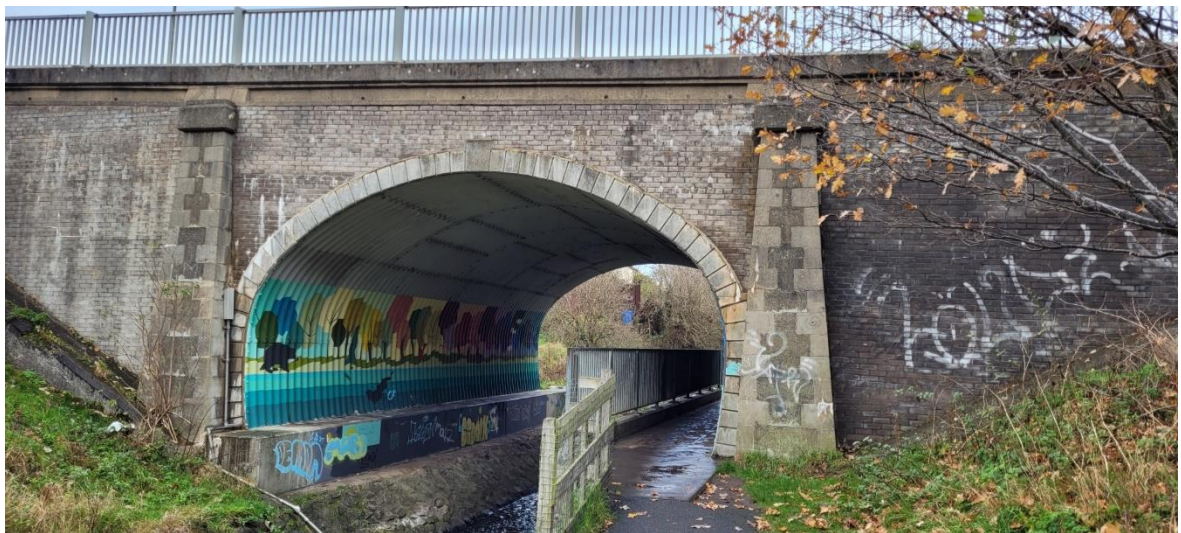
Figure 5 - Gilmerton Dykes Street (Hyvots Bank) Bridge
