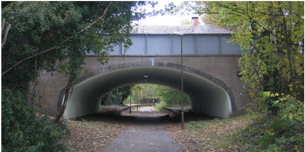
Figure 4 - Traquair Park East Bridge – Pinkhill
