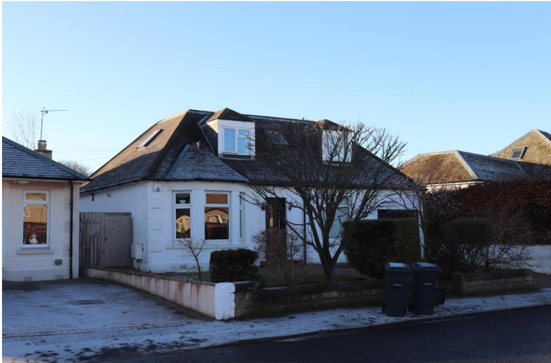
This property has a mansard extension to the main roof to the front and also a lower mansard roof over a later projecting extension to the rear. The first floor extends across the garage on one side.
