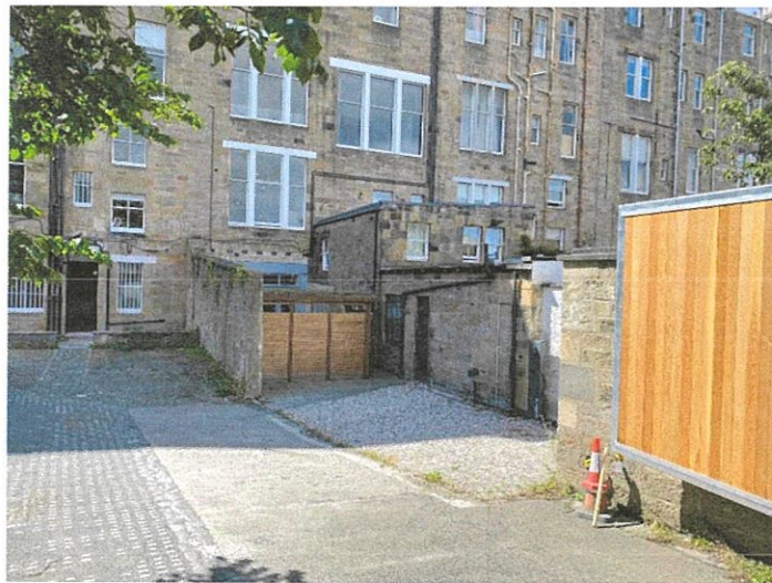
Rear View showing existing wing walls that conceal development
