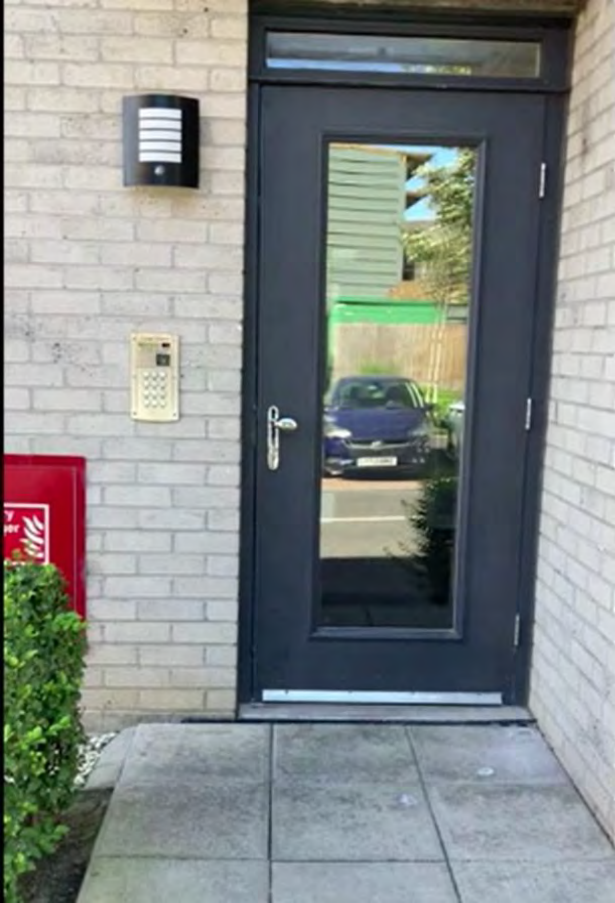
Entrance at street level to common stairway with entry phone.
